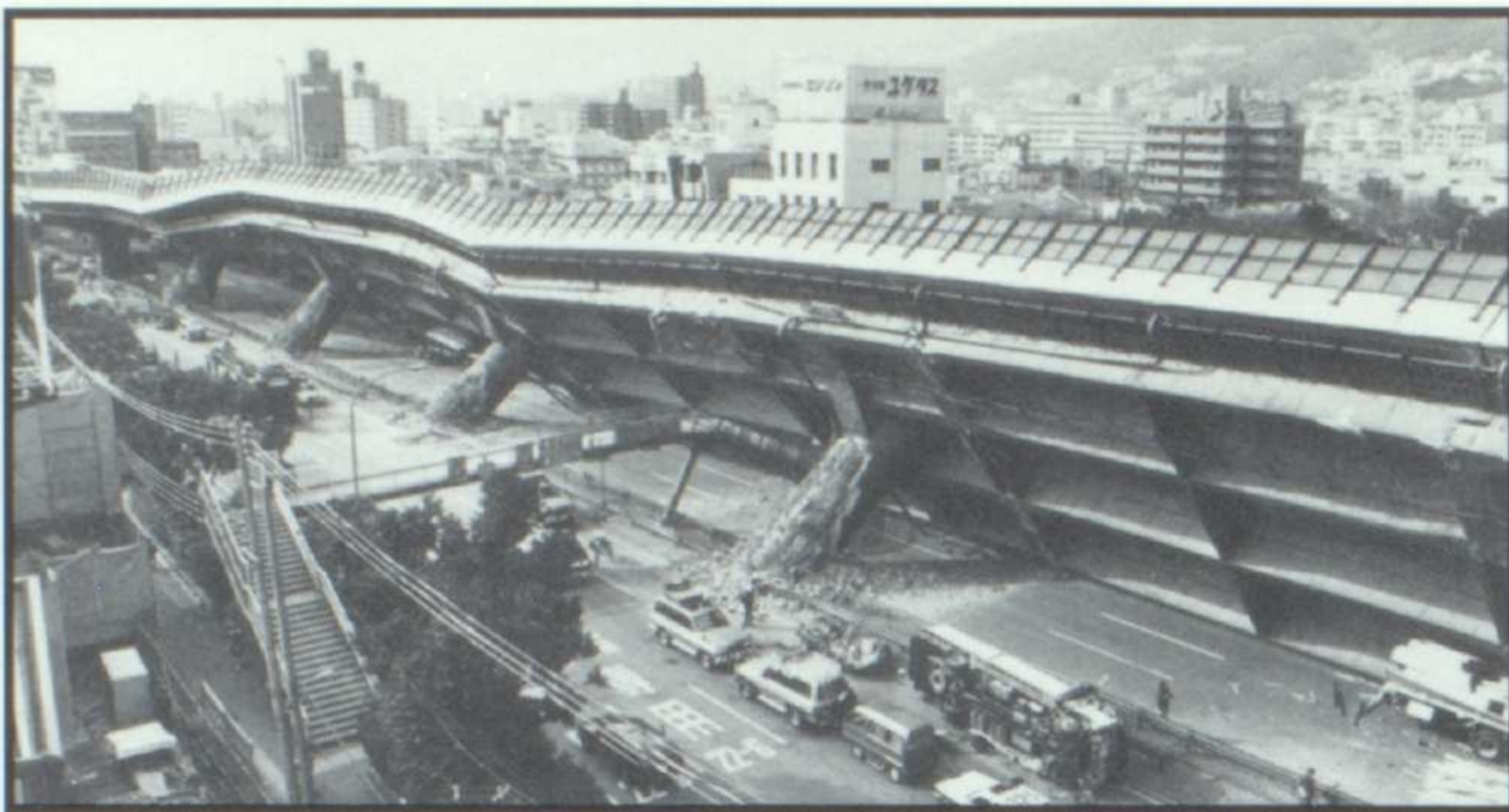
Powerful earthquakes tore through several western cities in Japan, toppling hundreds of buildings, touching off raging fires, and killing more than 5000 people.
