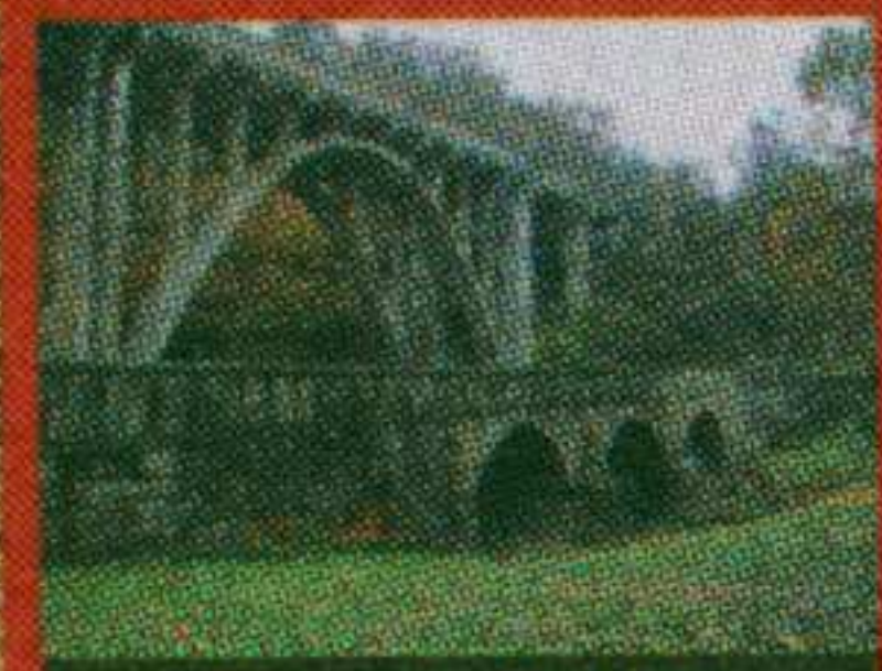
Blaines Bridge Belmont County
